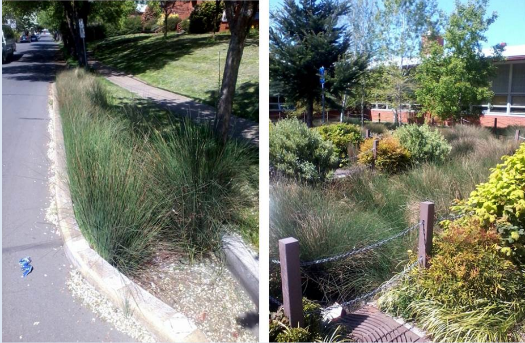
Figure 82. Street Gardens and Community Green Space Accept Runoff from Disconnected Roof Downspouts in Portland, Oregon
